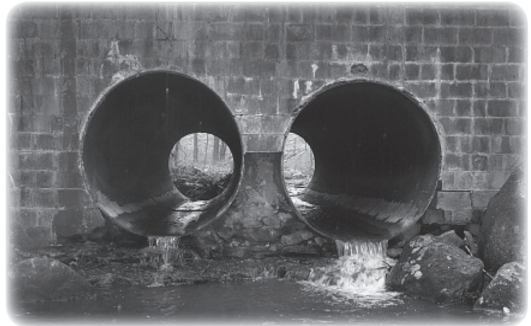
Figure 1. Example of culverts perched above streambed blocking fish passage.
